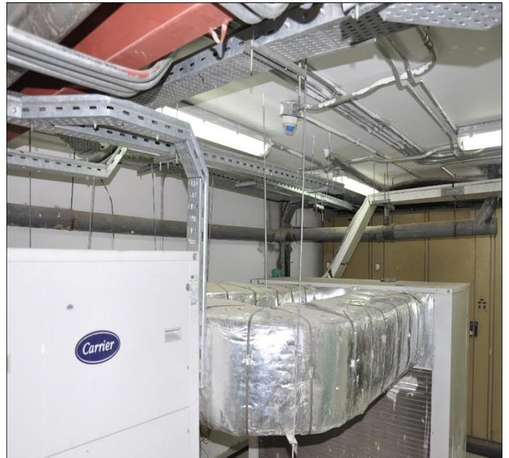
2. Split concealed AC units of various capacities: 30 AC units, supplied and installed by NeXTeP Construction, installation includes evaporator, condenser, grilles, hangers, supports and insulation work.
